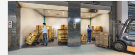
Massive goods lifts
