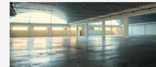
Top floor with Proflex roof
